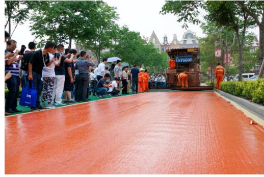
On-site construction demonstration of Colored Micro-surfacing
