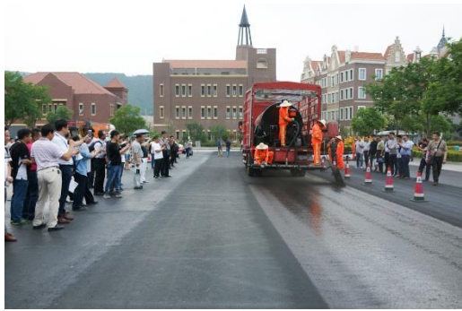
On-site construction demonstration of Micro-surfacing
