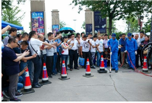
Live demonstration of Crack Sealing
